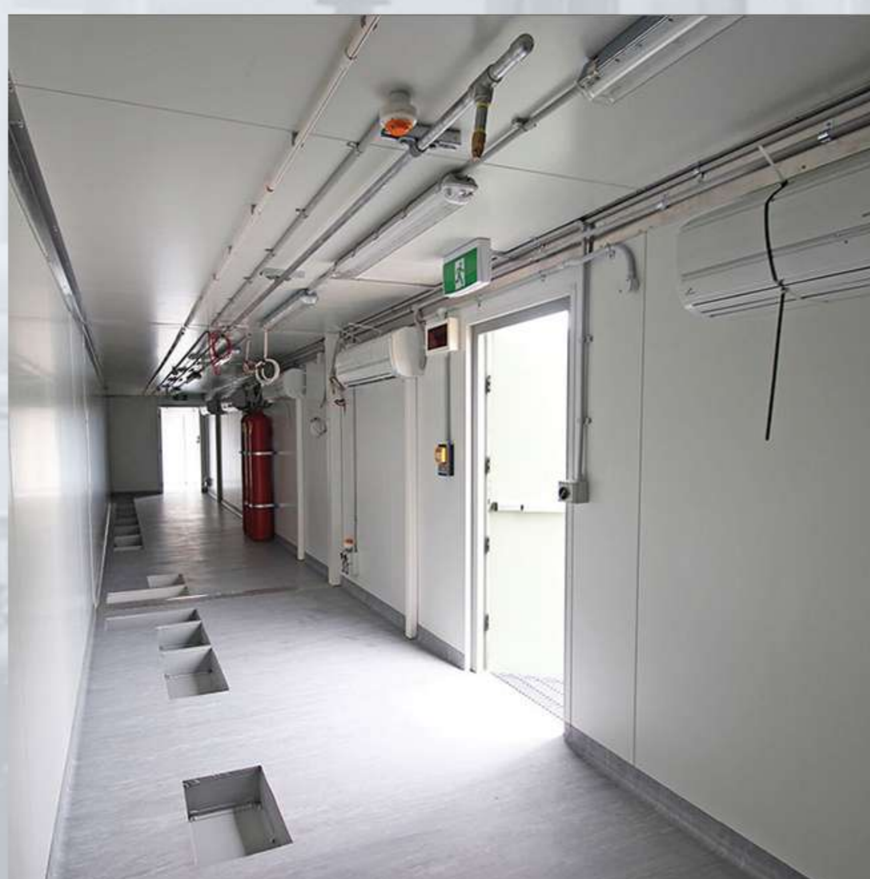
Pre-fabricated control substation container
